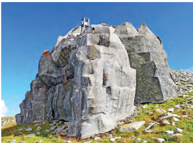
Fort Gütsch: From the evidence of the concealed casemate on the left-hand side, this elaborately camouflaged structure was probably a machine-gun bunker
